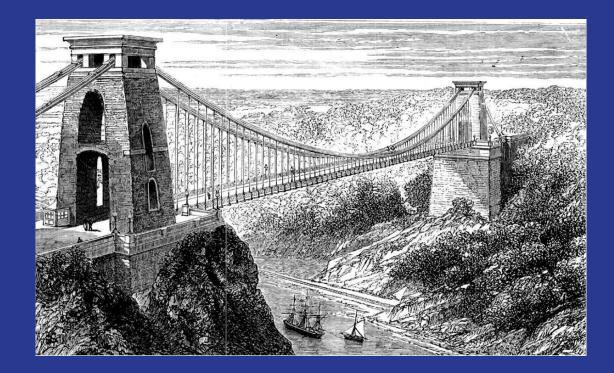
70. Suspension bridge cables hang in parabolas The suspension bridge cable shown in the accompanying figure supports a uniform load of w pounds per horizontal foot. It can be shown that if H is the horizontal tension of the cable at the origin, then the curve of the cable satisfies the equation
